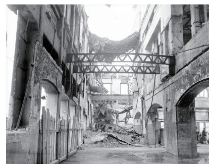
View from inside Hiroshima Station looking southeast. The main waiting room is on the right and the platform is on the left. The roof and second floor of this section have collapsed. (Photo taken by the U.S. Army on November 18, 1945, courtesy of Hiroshima Peace Memorial Museum)
